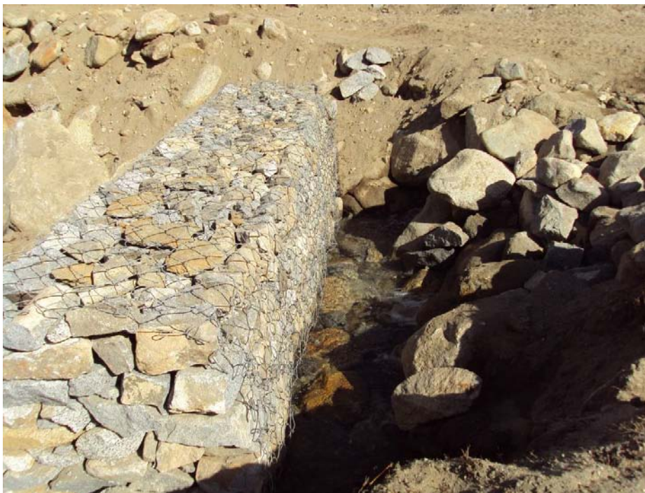
Figure 14: Close-up of Dam-and-Gate system diverting Water into the Artificial Canal
