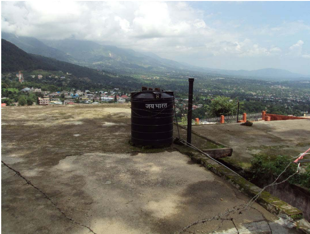
Figure 6: A Roof-top Storage Tank in a Household with a Private Water Connection
