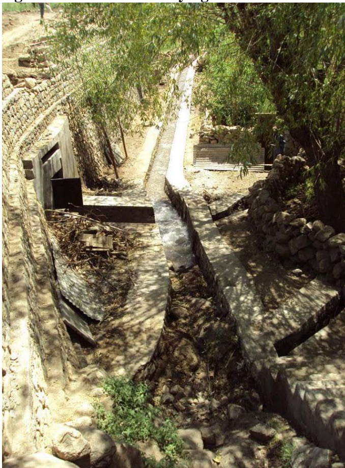
Figure 18: Channel conveying Water from Pond to Farmlands
